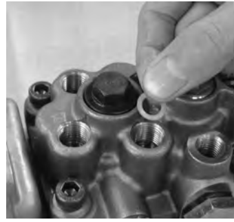
Install the new packing, (delivery valve seat).
